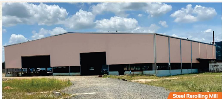
Steel Rerolling Mill
